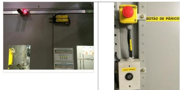
Figure 9: Experimental Hutch Door and Interlock Control Box
